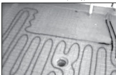
Wet Area on mesh and membrane
