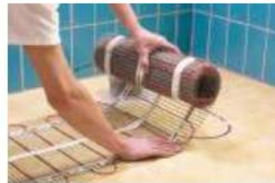
5. Check the heating mat cable resistance and its insulation resistance values. Roll out the mat onto the floor from the thermostat position, sticky side down.
