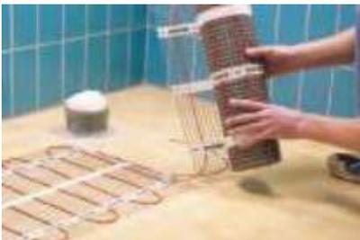
7. **Space** 100 mm from walls. Avoid any obstacles and fixtures. Mats spaced approx. 80mm apart. Minimum spacing 50mm between any two heating elements.
