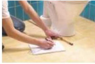
2. **Draw a plan** showing the actual heated area, heating mat, cold tail location, floor sensor position, thermostat and connection box (if any).
