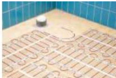
8. **Lay out mat** to entire surface. Check the cable resistance and the insulation resistance values again before laying tiles. Photograph installation layout and meter readings.
