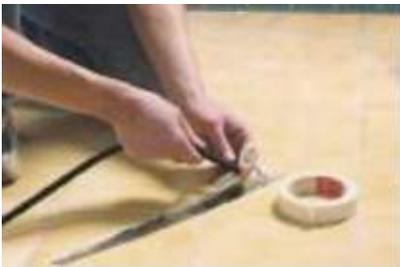
4. Install flexible **sensor conduit** (10mm OD) into the groove. Grooves are also needed for the terminations. Clean the floor so there is no dust or sharp protrusions.
