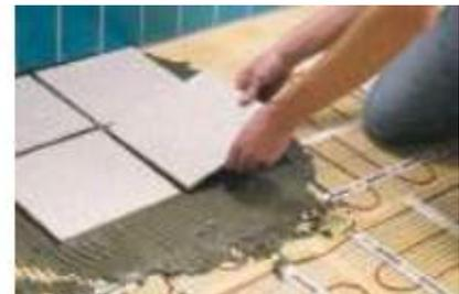
9. Apply tile **glue and lay tiles**. Careful not to damage the cables. Check the cable resistance and the insulation resistance values again when installing the thermostat.
