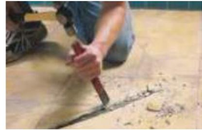
3. Glue appropriate **thermal insulation** onto the existing floor (e.g. F-Board). Allow to dry (min 24 hr). Cut a groove for sensor and terminations.
