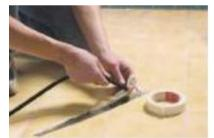
Install flexible sensor conduit (10mm OD) into the groove. Grooves are also needed for the terminations. Clean the floor so there is no dust or sharp protrusions.
