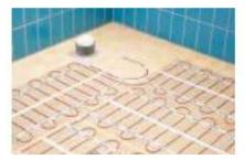
8. Lay out mat to entire surface. Check the cable resistance and the insulation resistance values again before laying tiles. Photograph installation layout and meter readings.
