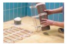
Space 100 mm from walls. Avoid any obstacles and fixtures. Mats spaced approx. 80mm apart. Minimum spacing 50mm between any two heating elements.
