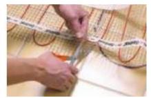
6. The mesh mat can be cut to go around fixtures and to cover the floor area to be heated. DO NOT CUT the heating element.
