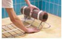
Check the heating mat cable resistance and its insulation resistance values. Roll out the mat onto the floor from the thermostat position, sticky side down.
