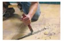
Glue appropriate thermal insulation onto the existing floor (e.g. F-Board). Allow to dry (min 24 hr). Cut a groove for sensor and terminations.
