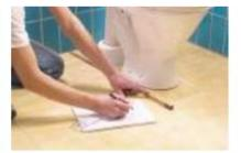
2. Draw a plan showing the actual heated area, heating mat, cold tail location, floor sensor position, thermostat and connection box (if any).
